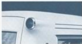
NEW TUNNEL LIGHTS are designed as an integral part of the roof.
