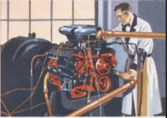
ANOTHER set of accurate instruments carried on the "bicycle wheel." Here, fuel economy is being measured to give the engineers another "picture" of performance.
